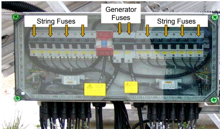
Fig. A6 - Array junction box
